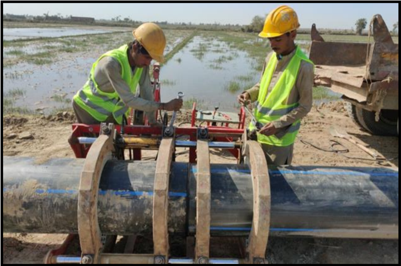
WW-12 (Zone-C) Jointing of the 500mm dia pipe for Rising main work is in progress at Shamb-e-Shah to Noorwah Jacobabad
