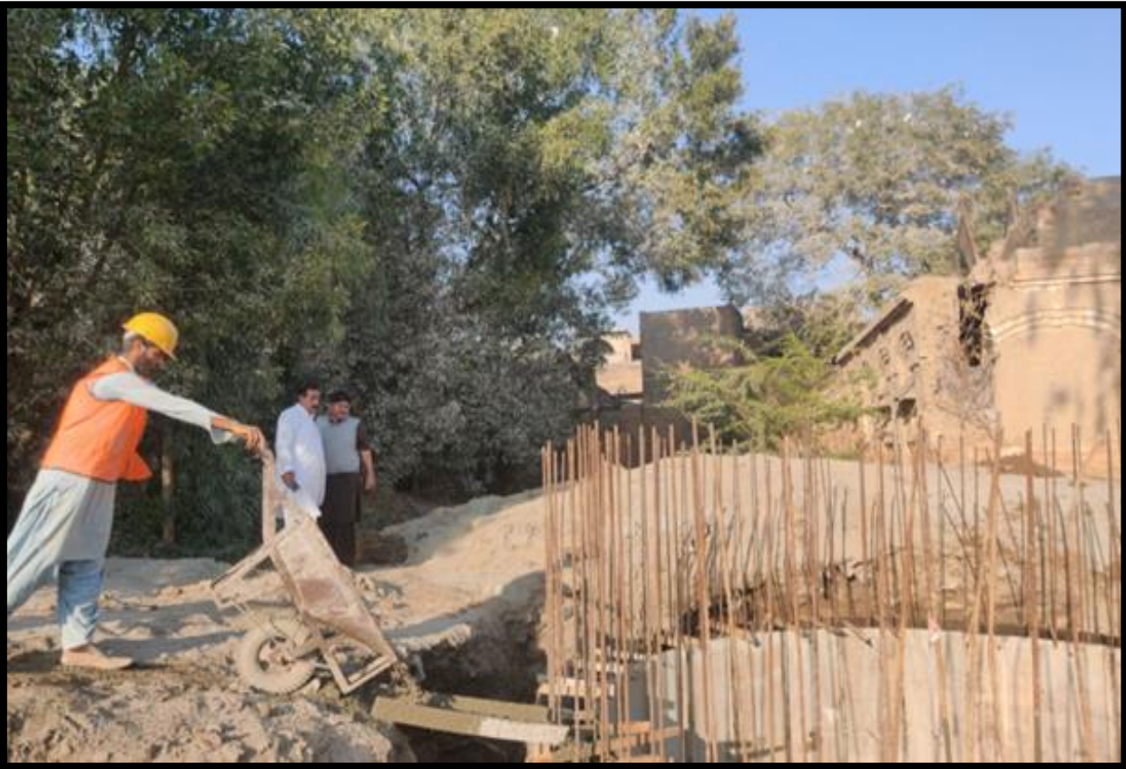
WW-09 (Zone-C) Concrete pouring of sump wall work is in progress Railway Station Jacobabad
