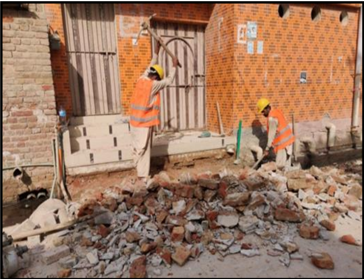
WW-07 (Zone-A) Dismantling & Excavation work is progress
