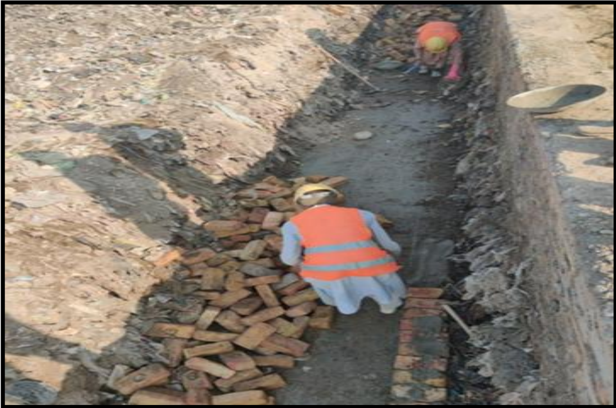
WW-08 (Zone-B) Brick masonry of drain work is in progress at street No. 1-E8 Al Murtaza Colony Jacobabad
