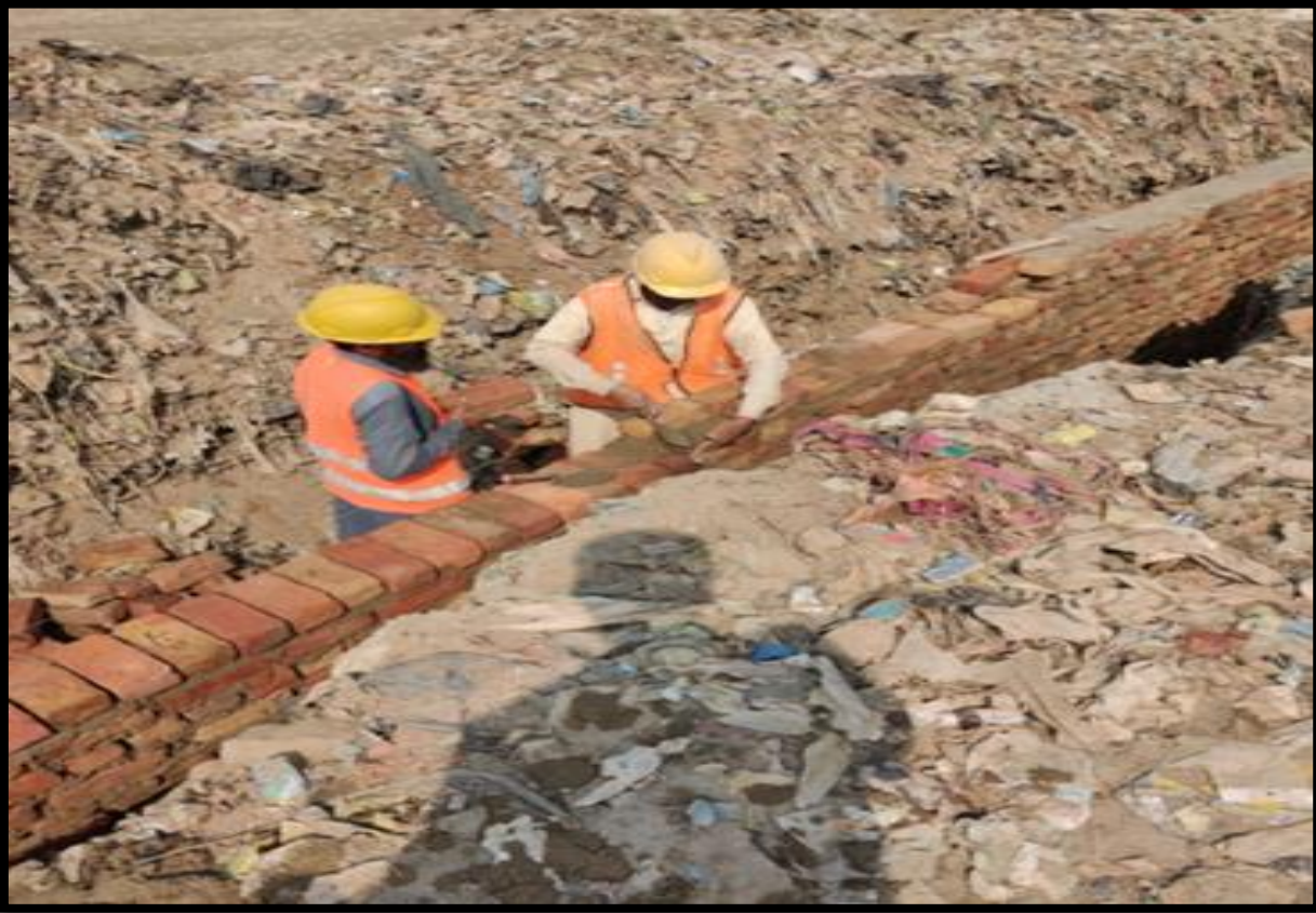
WW-08 (Zone-B) Brick masonry of drain work is in progress at street No. 1E8 Al Murtaza Colony Jacobabad
