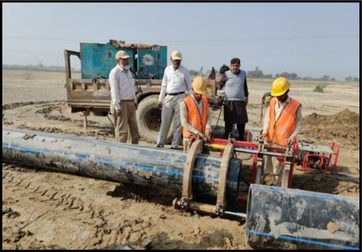
WW-12 (Zone-C) Jointing of the 500mm dia pipe for Rising main work is in progress at Shamb-e-Shah to Noorwah Jacobabad
