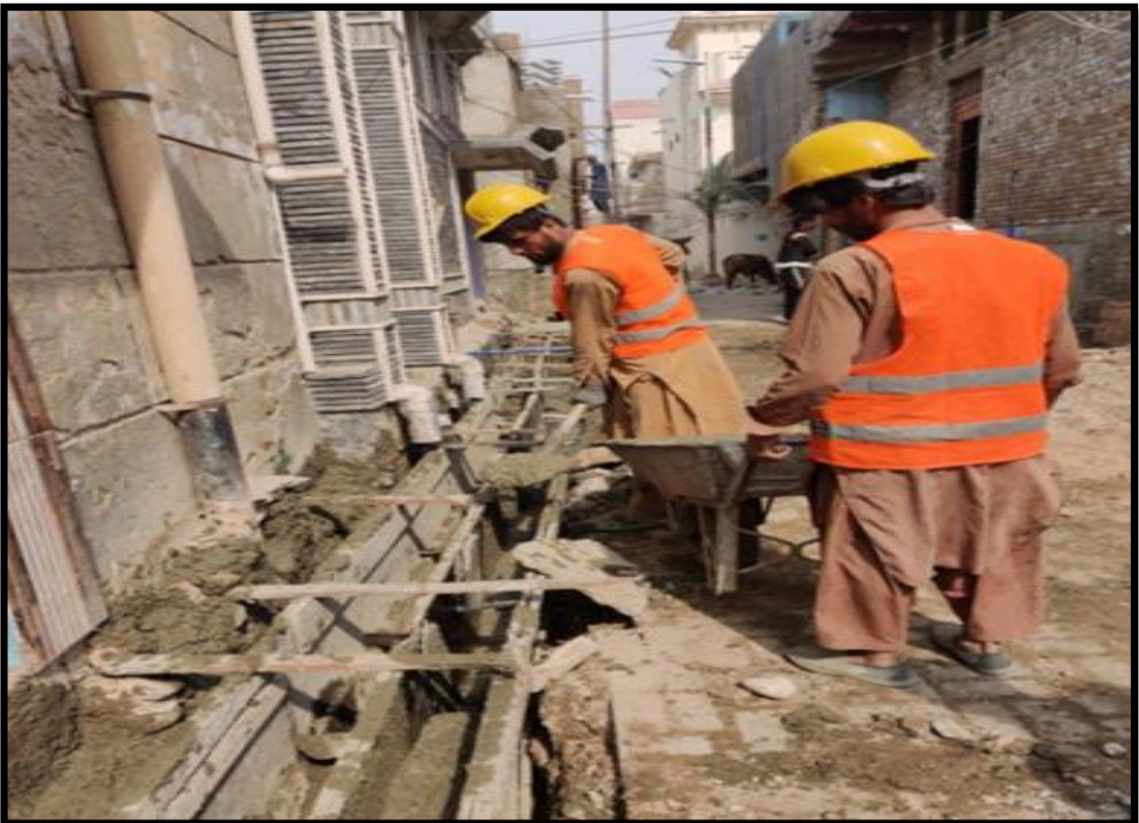
WW-07 (Zone-A) Concrete pouring of drain wall work in progress
