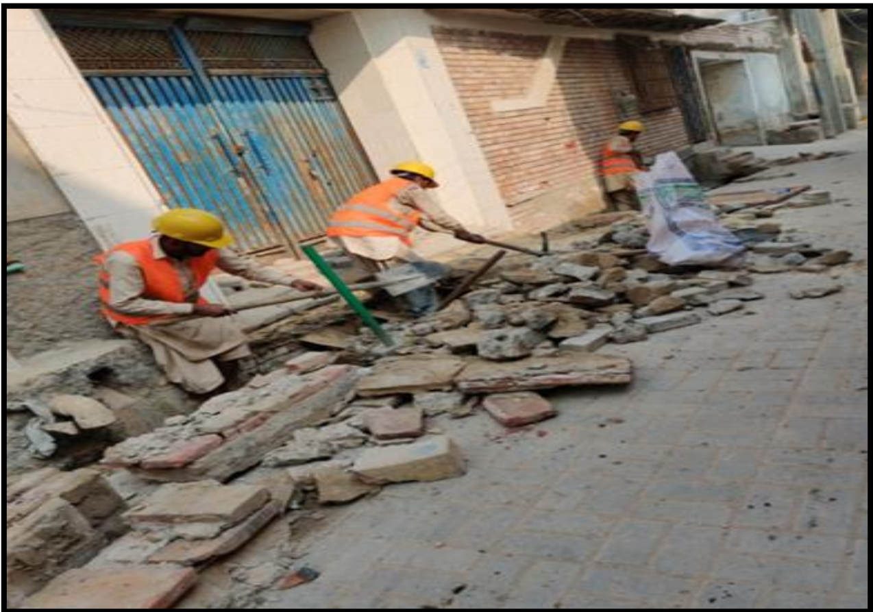
WW-07 (Zone-A) Dismantling work is in progress
