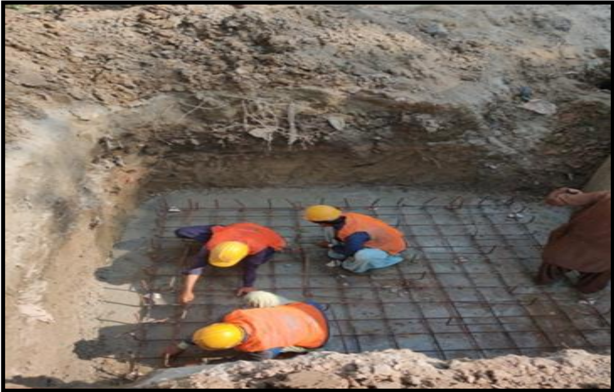
WW-09 (Zone-C) Reinforcement of Screen Chamber work is progress at Railway Station Jacobabad
