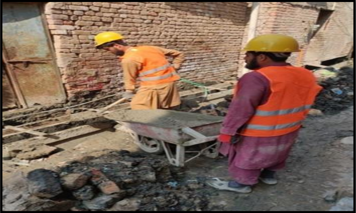
WW-07 (Zone-A) Concrete pouring of drain wall work in progress
