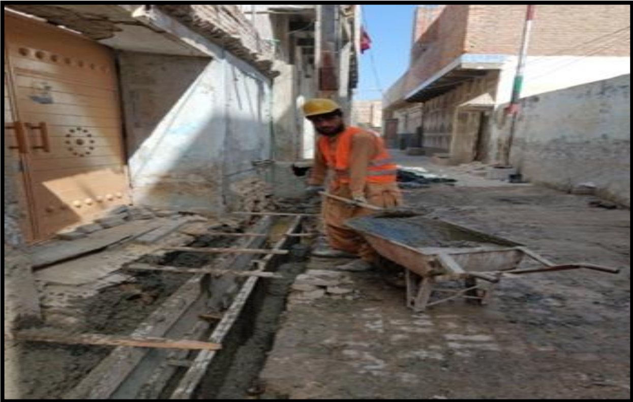
WW-07 (Zone-A) Concrete pouring of drain wall work is in progress
