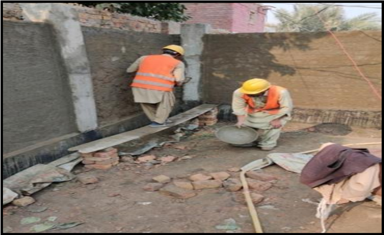
WW-07 (Zone-A) Plaster of boundary wall work is in progress at Revenue Colony Jacobabad
