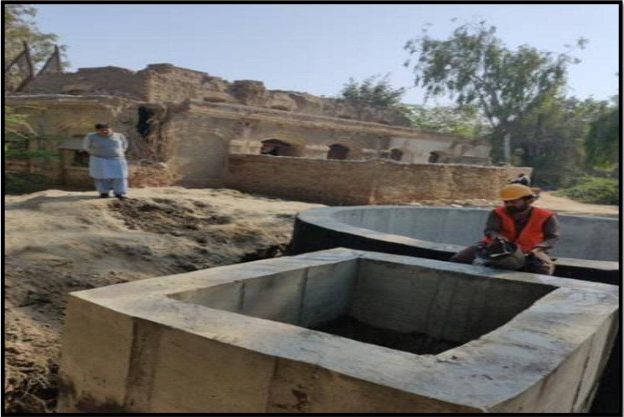
WW-09 (Zone-C) Water Curing of Sump work is in progress at Railway Station Jacobabad
