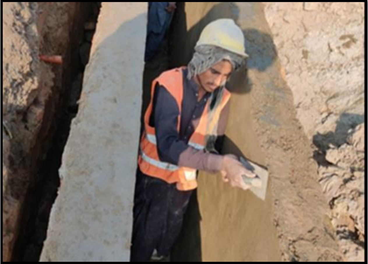
WW-08 (Zone-B) Plaster of drain work in progress at Street No. 11-A, Al Murtaza Colony Jacobabad
