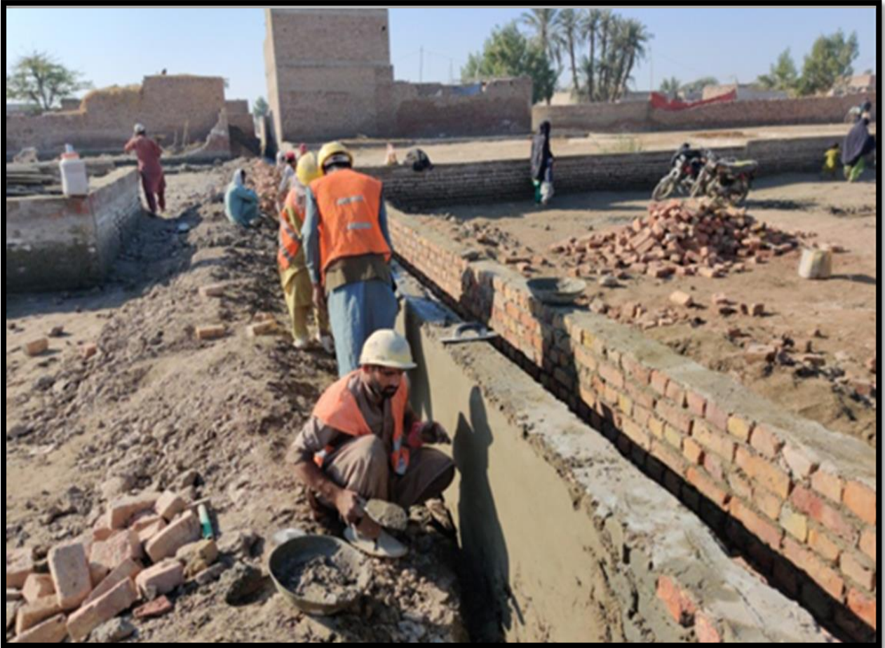
WW-08 (Zone-B) Plaster of Brick Masonry of drain work in progress at street No. 13-D Al Murtaza Colony Jacobabad
