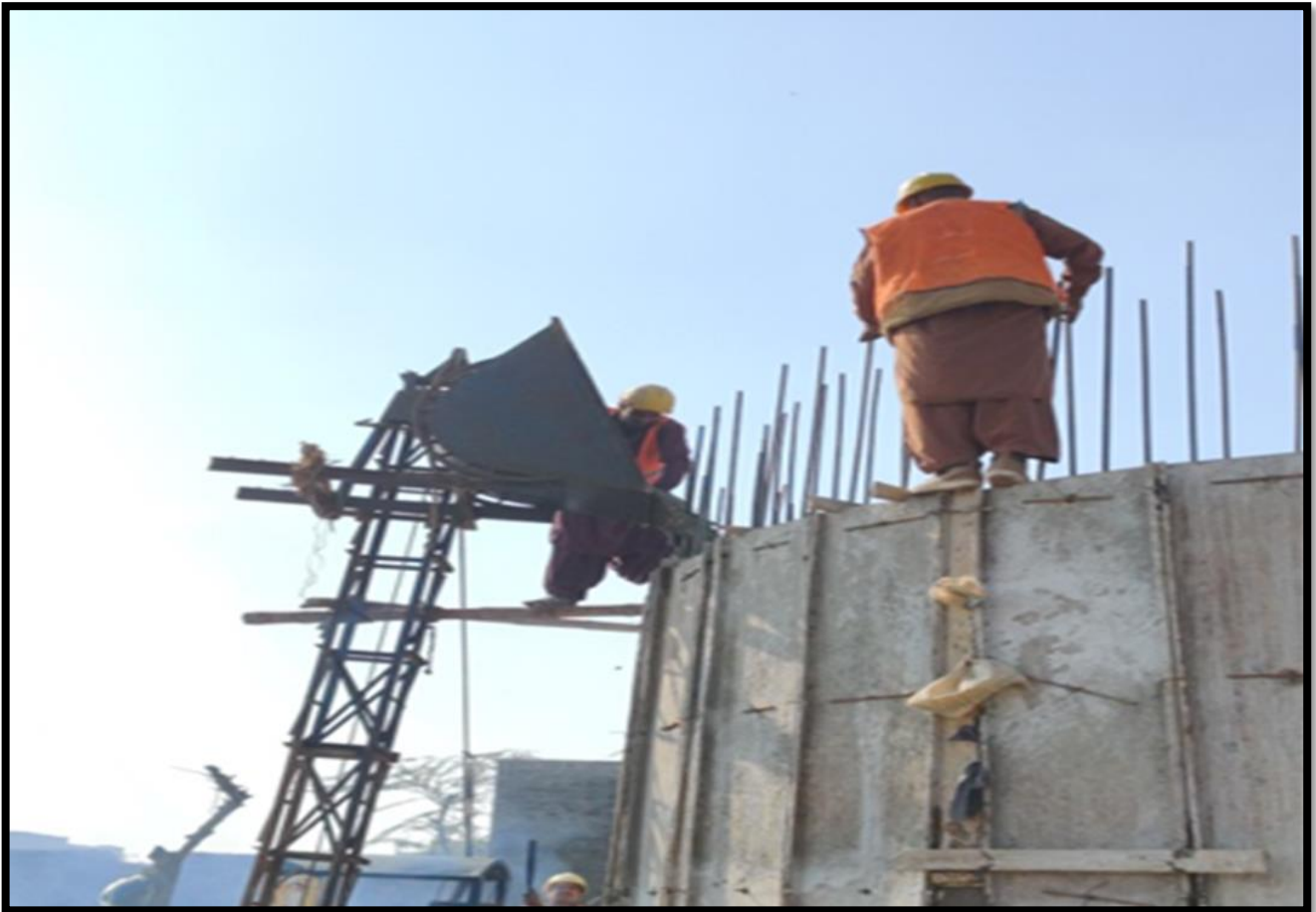
WW-08 (Zone-B) Concrete Pouring of Sump wall in progress at A Al Murtaza Colony Jacobabad
