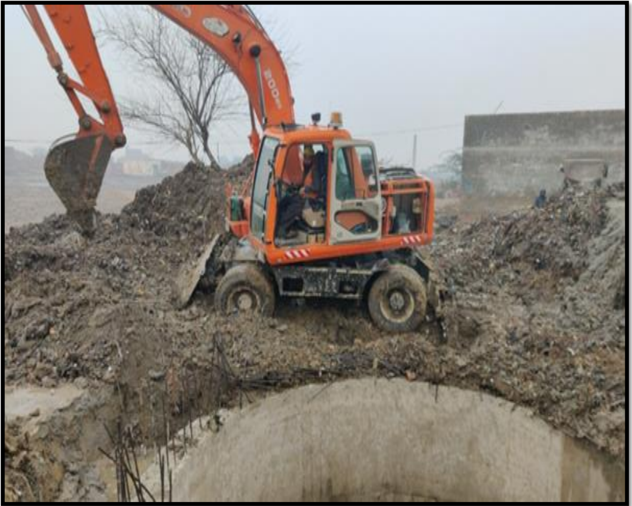
WW-08 (Zone-B) Sinking the Sump work in progress with the help of Excavator at Al Murtaza Colony Jacobabad
