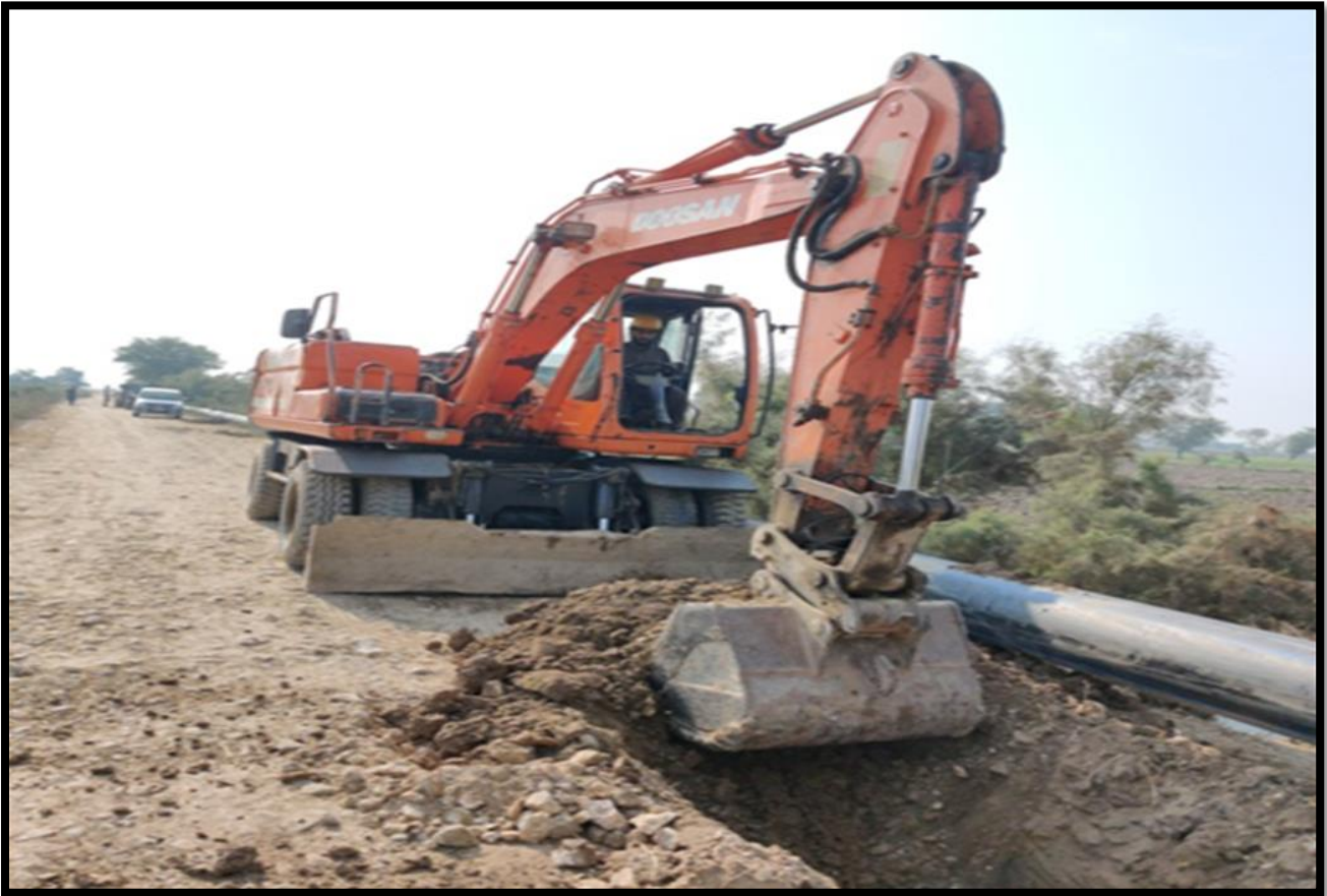
WW-12 (Zone-C) Excavation for lying HDPE 500mm diameter Pipe for Raising Main work in progress at Shamb-e-Shah to Noor Wah
