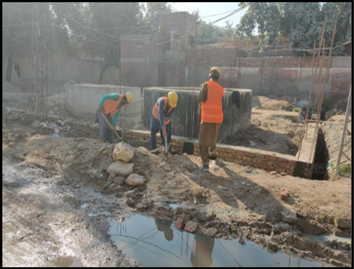
WW-07 (Zone-A) Back filling of Boundary wall work in progress at Revenue Colony Jacobabad
