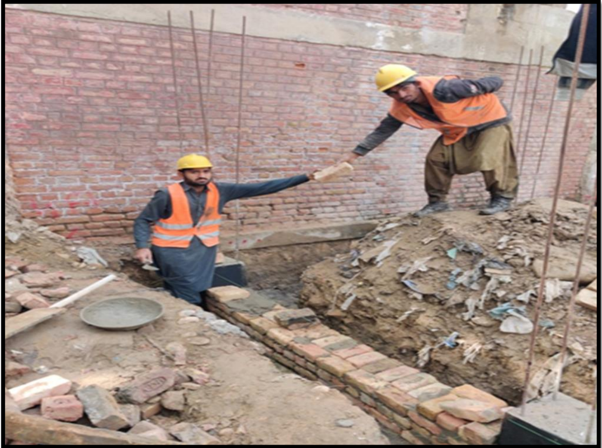
WW-07 (Zone-B) Brick Masonry of Boundary wall work in progress at Revenue colony PS Jacobabad
