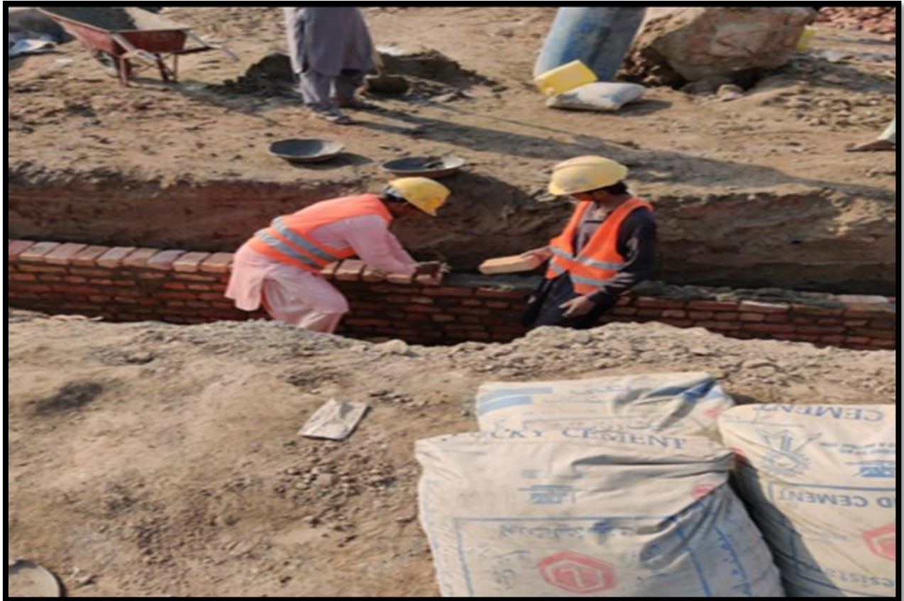
WW-08 (Zone B) Brick Masonry of drain work in progress at Al Murtaza Colony Jacobabad
