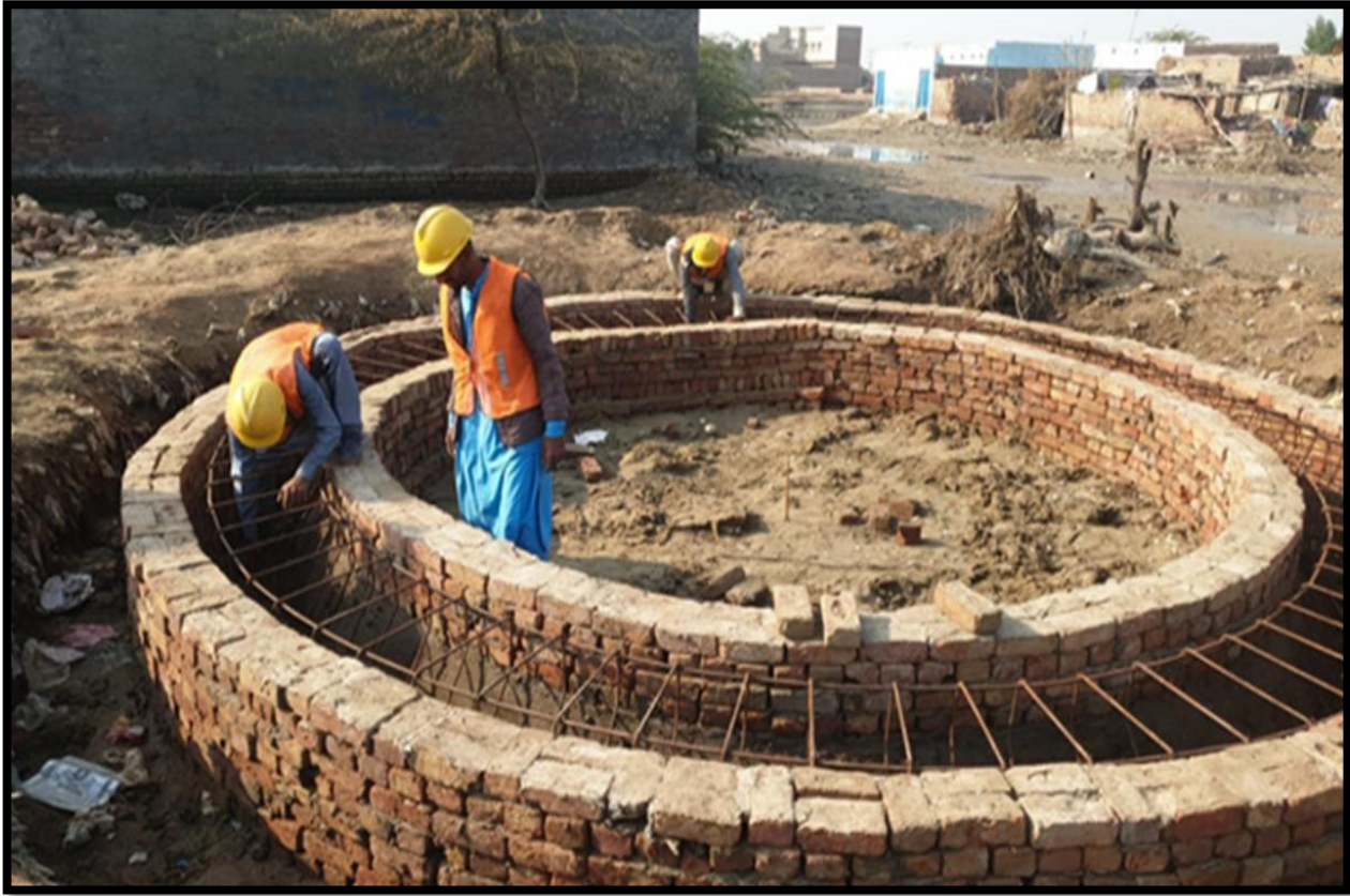
WW-08 (Zone-B) Steel Fixing Reinforcement Sump work is in progress at Al Murtaza Colony Jacobabad
