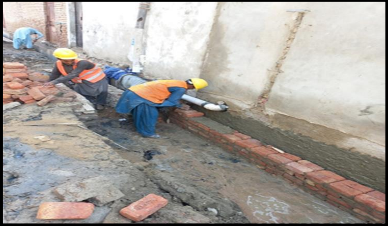
WW-08 (Zone-B) Brick Masonry of drain is in progress at street No. 4-A Al Murtaza Colony Jacobabad
