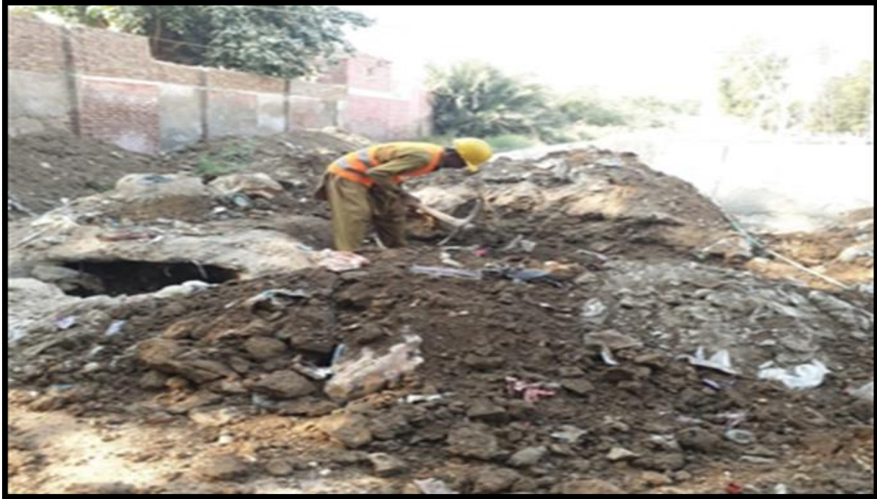
WW-07 (Zone-A) Excavation for Boundary wall of Revenue Colony disposal work is in progress
