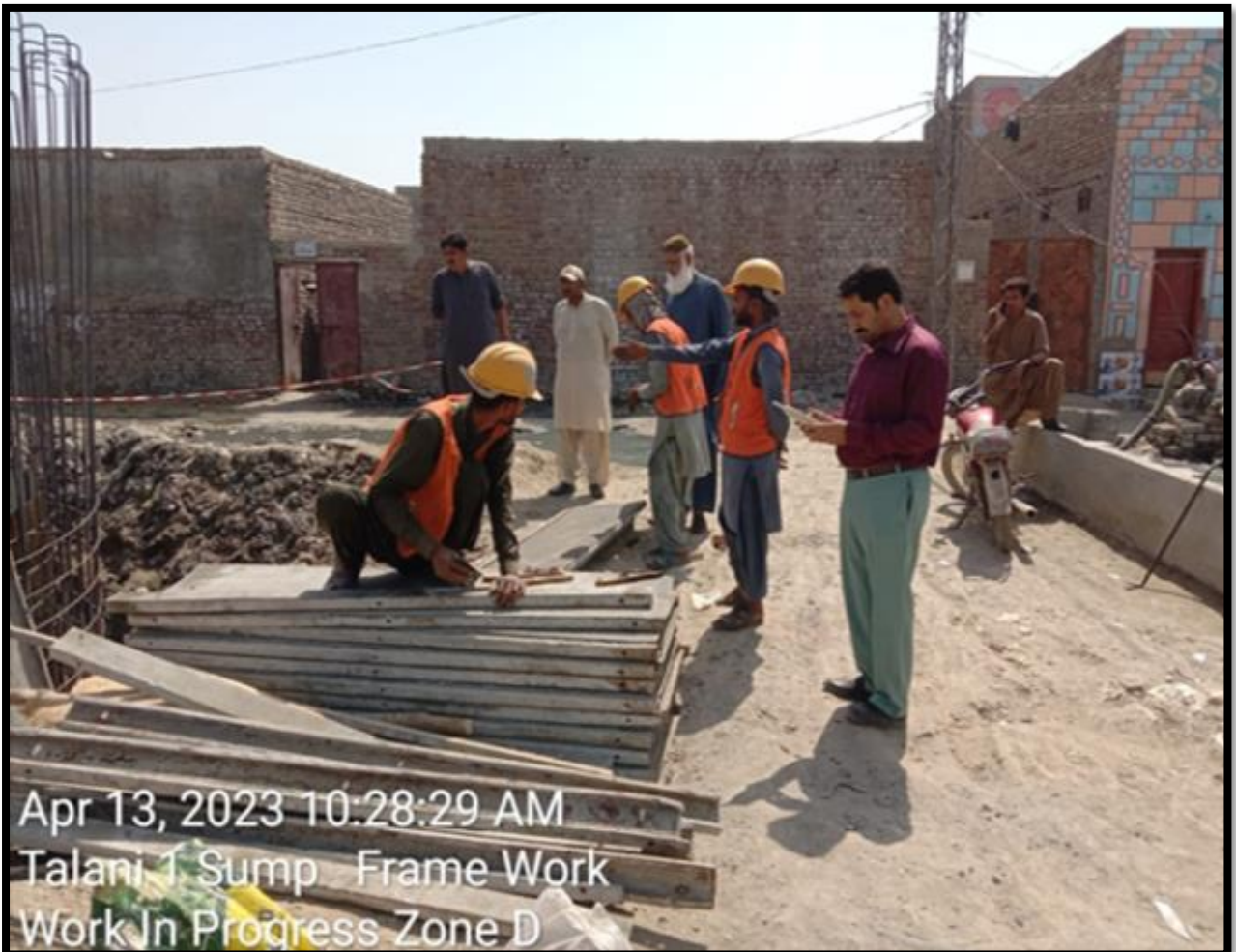
WW-10 (Zone-D) Reinforcement & Shuttering formwork of Talani-I Sump work in progress
