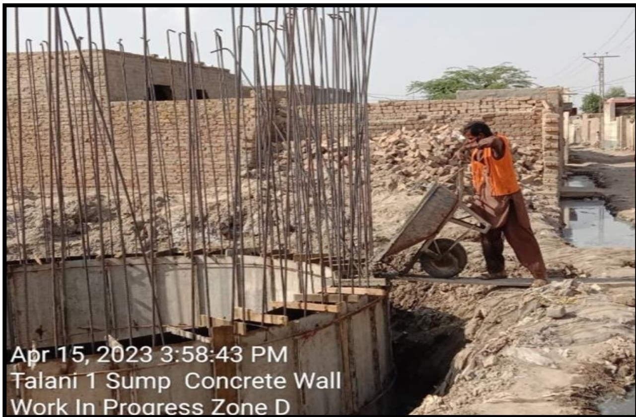
WW-10 (Zone D) Concrete pouring of Sump Talani-I work in progress
