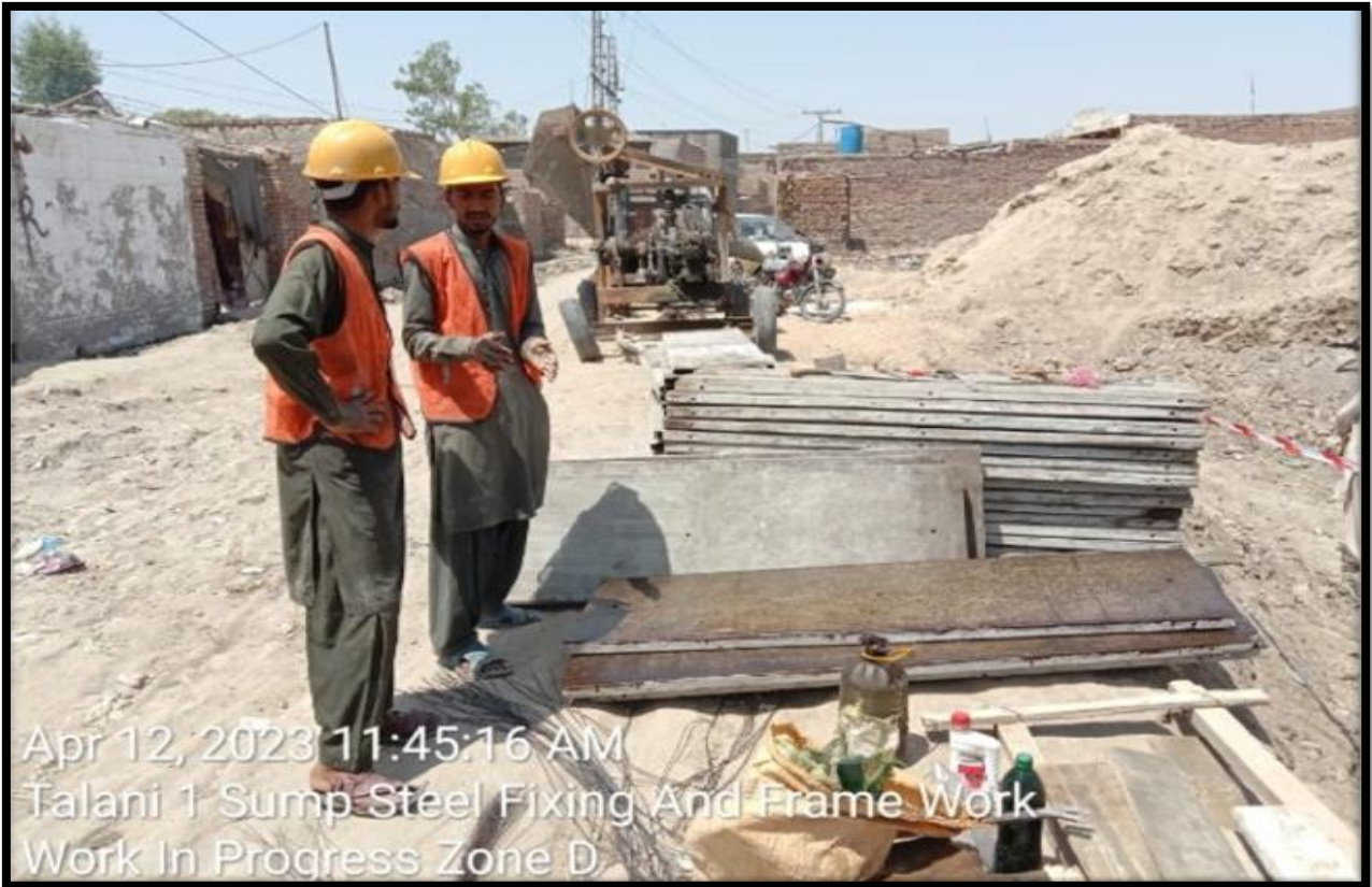
WW-10 (Zone-D) Shuttering formwork of Talani-I Sump work in progress
