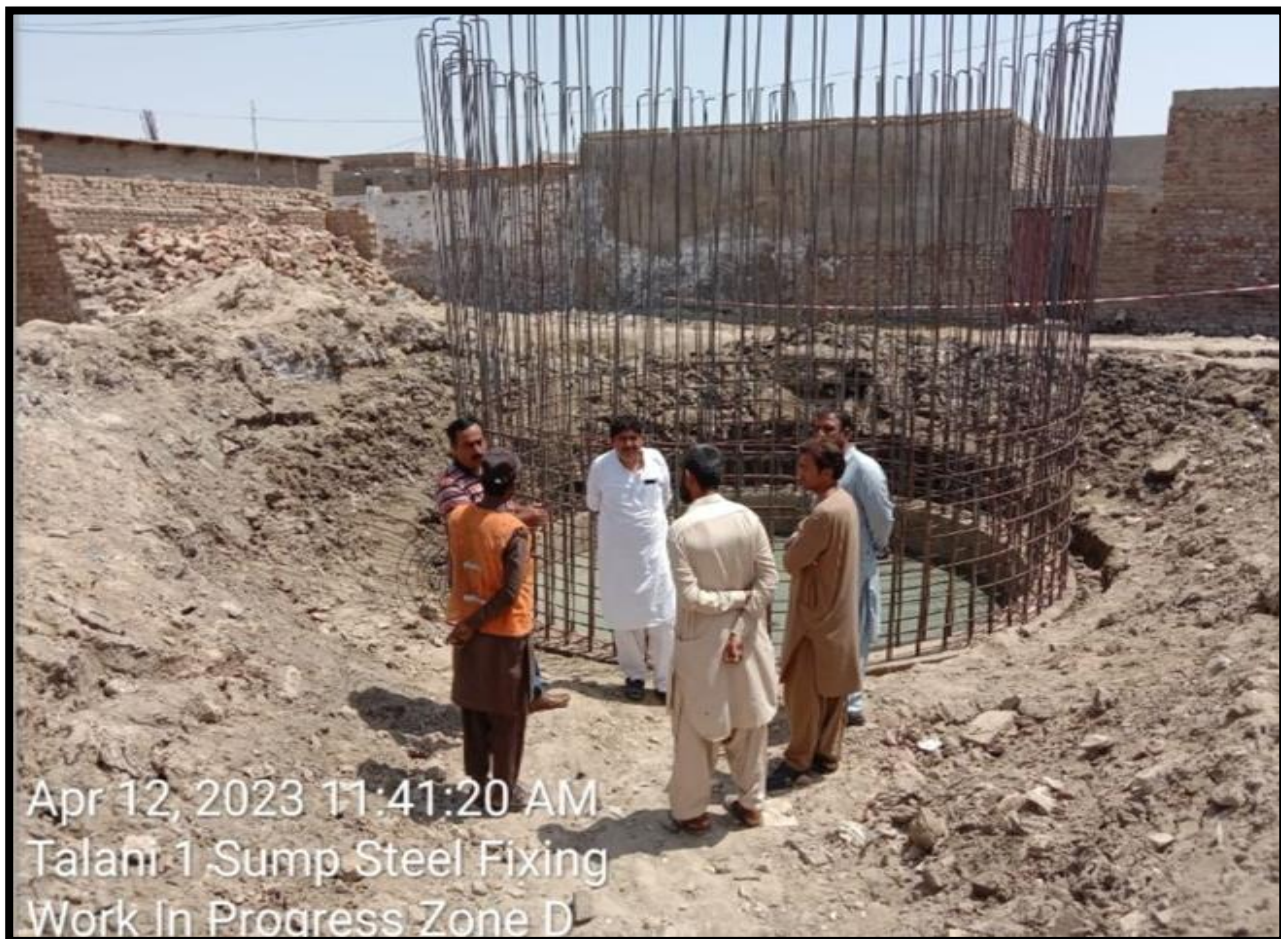
WW-10 (Zone-D) Reinforcement /steel fixing at Talani-I sump work in progress
