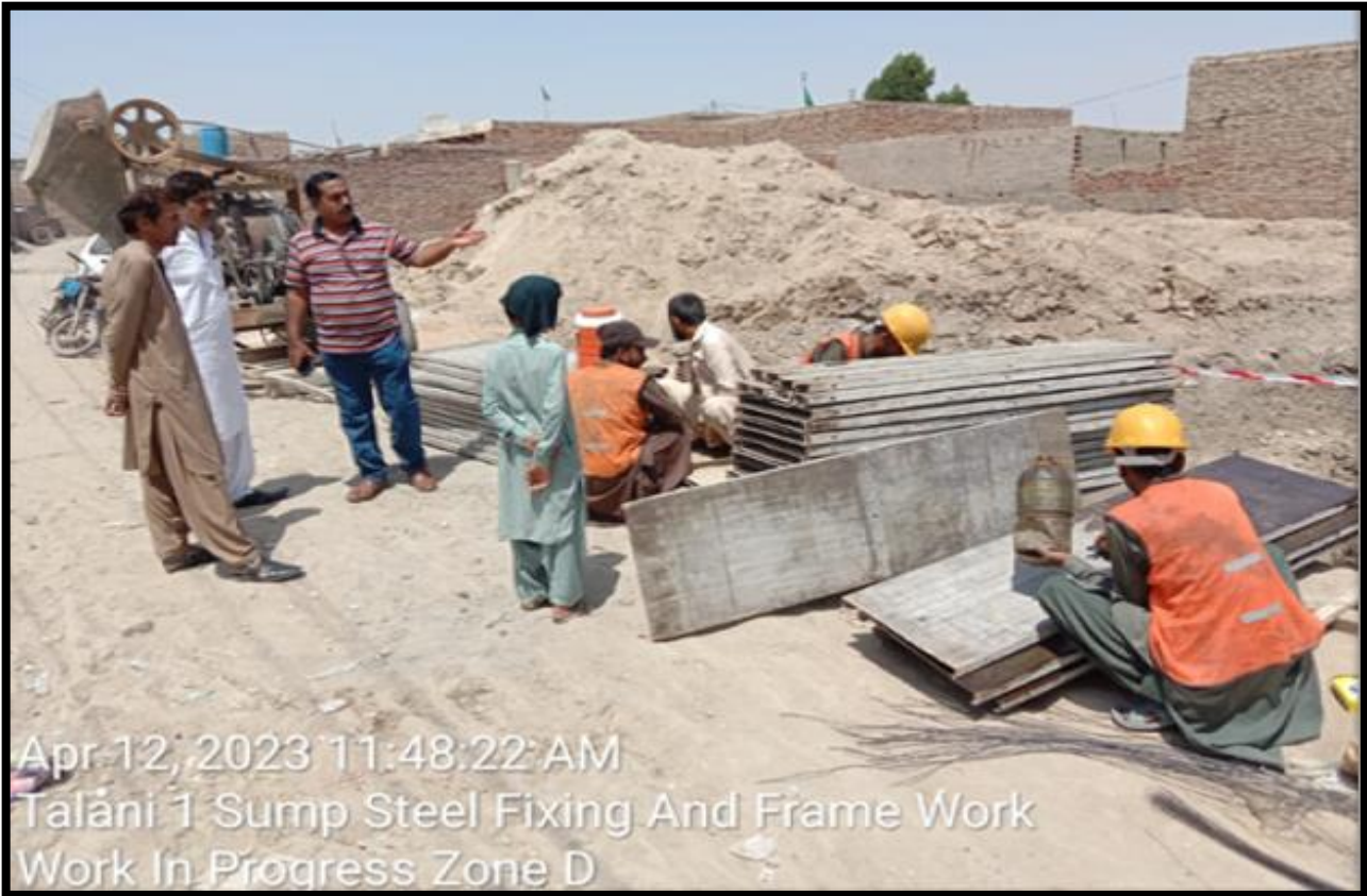
WW-10 (Zone-D) Shuttering formwork at Talani-I Sump work in progress
