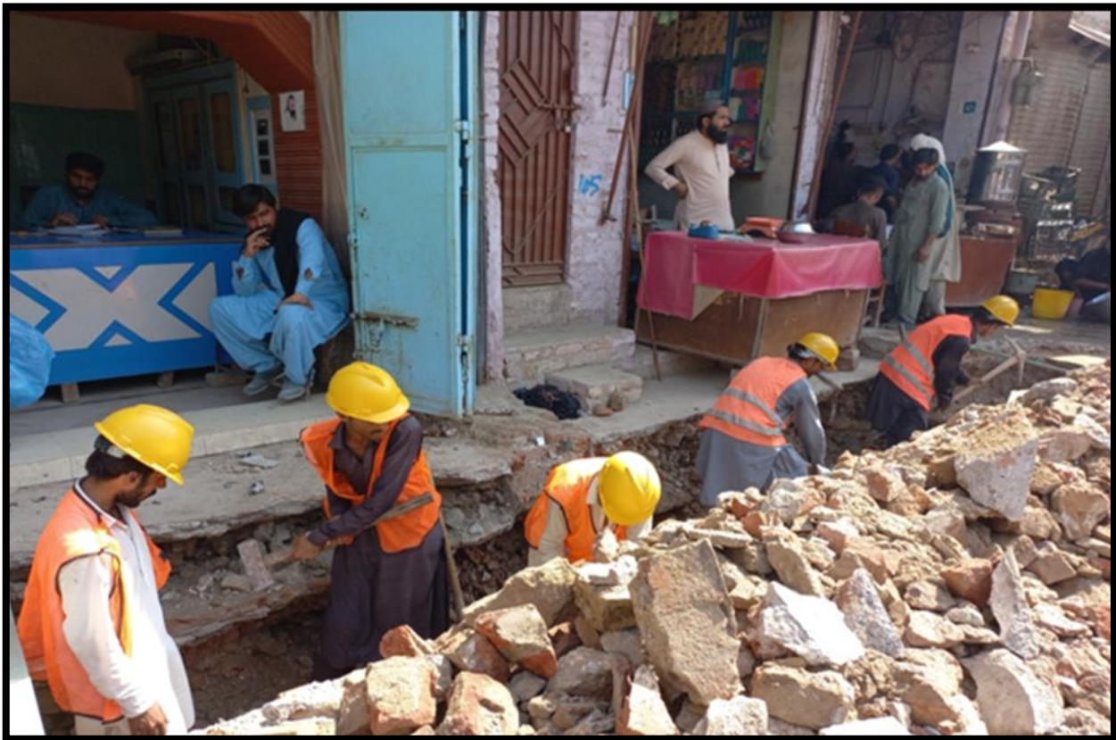
WW-08 (Zone-B) Excavation, dismantling work is in progress
