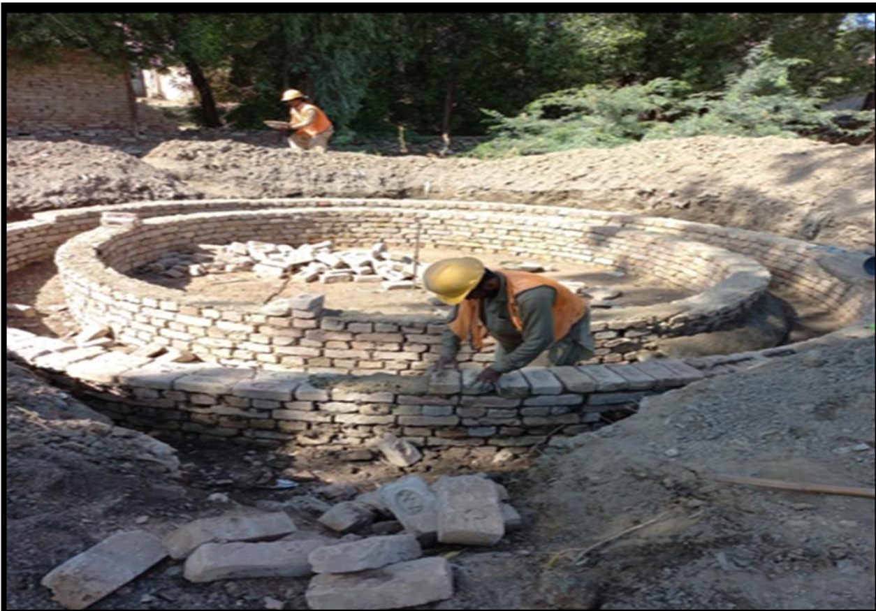
WW-09 (Zone-C) Sump of Railway Station work is in progress
