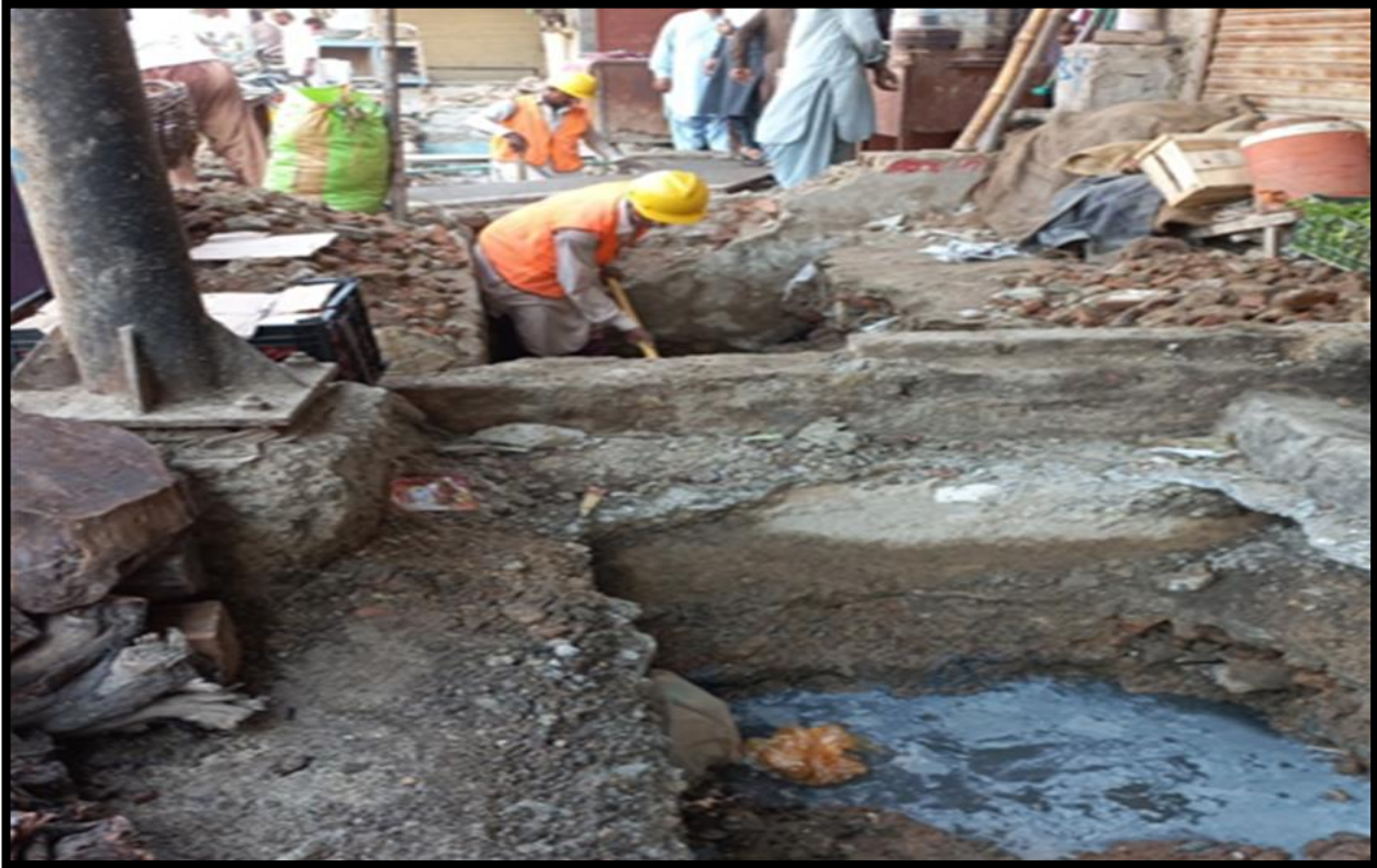
WW-08 (Zone-B) Excavation, dismantling work is in progress
