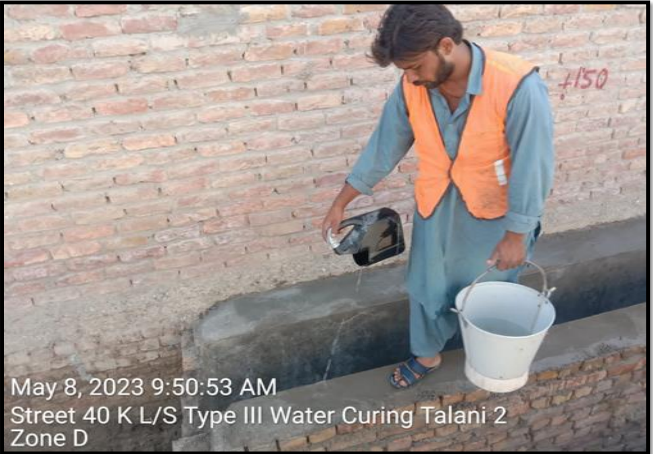
WW-10 (Zone-D) Water Curing of newly constructed Drain is in progress
