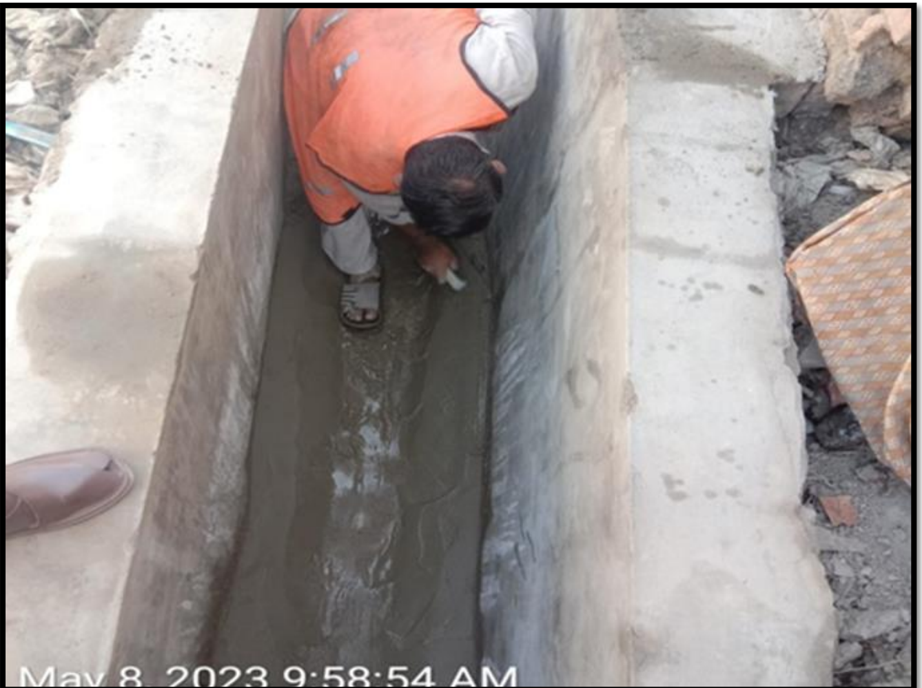
WW-10 (Zone-D) Plaster and Chamfer of Drain work is in progress
