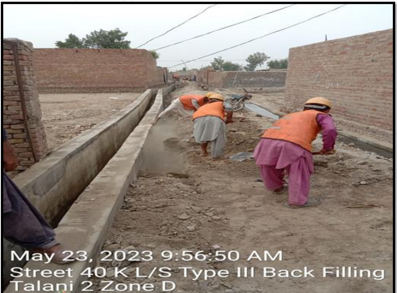
WW-10 (Zone-D) Backfilling of Drain work in progress
