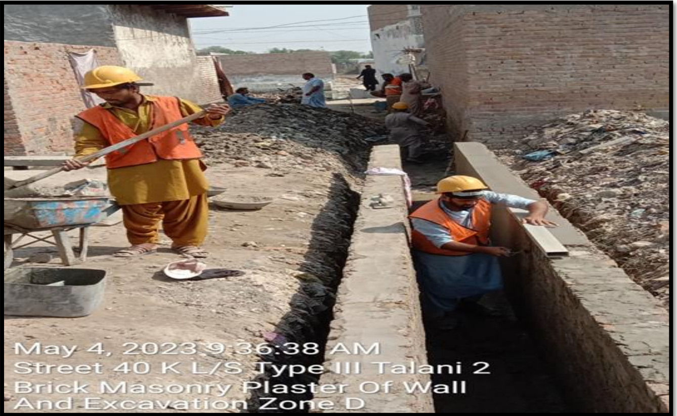
WW-10 (Zone-D) Plaster and Chamfer of Drain work is in progress
