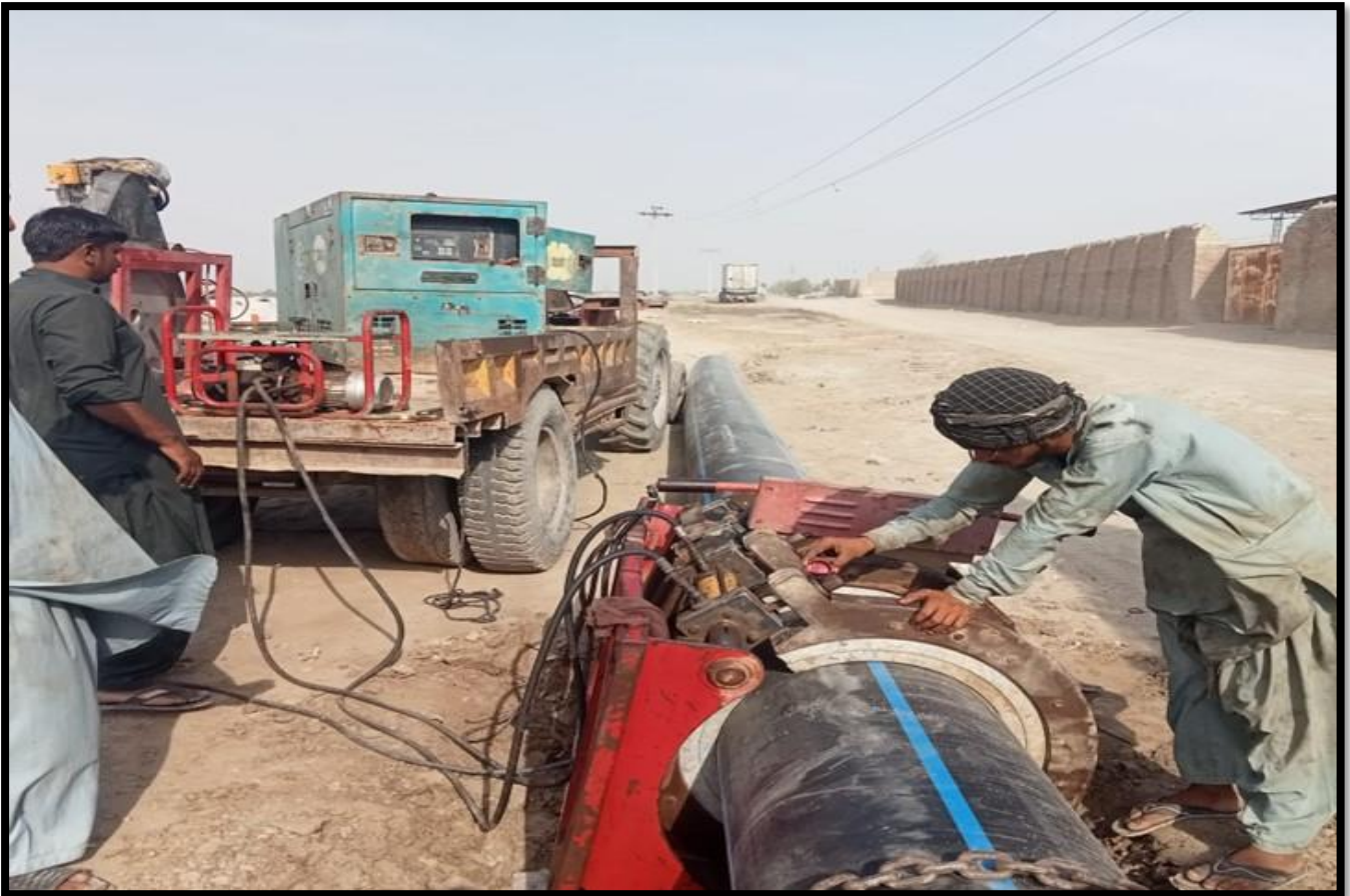
WW-12 (Zone-C) Jointing of 500mm diameter pipe Rising Main work is in progress
