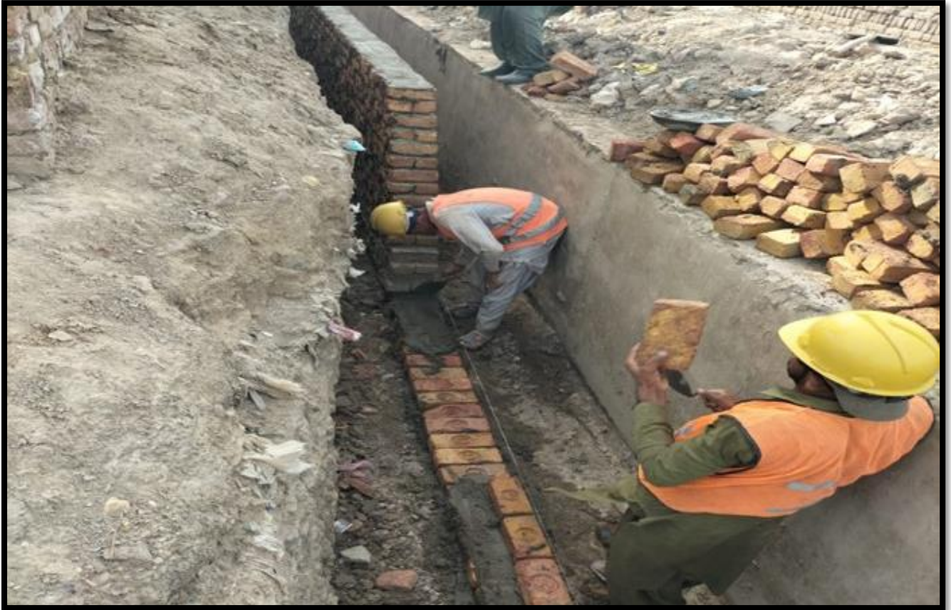
WW-08 (Zone-B) Brick Masonry of Drain Street No.11 A1 Al Murtaza Colony work is in progress
