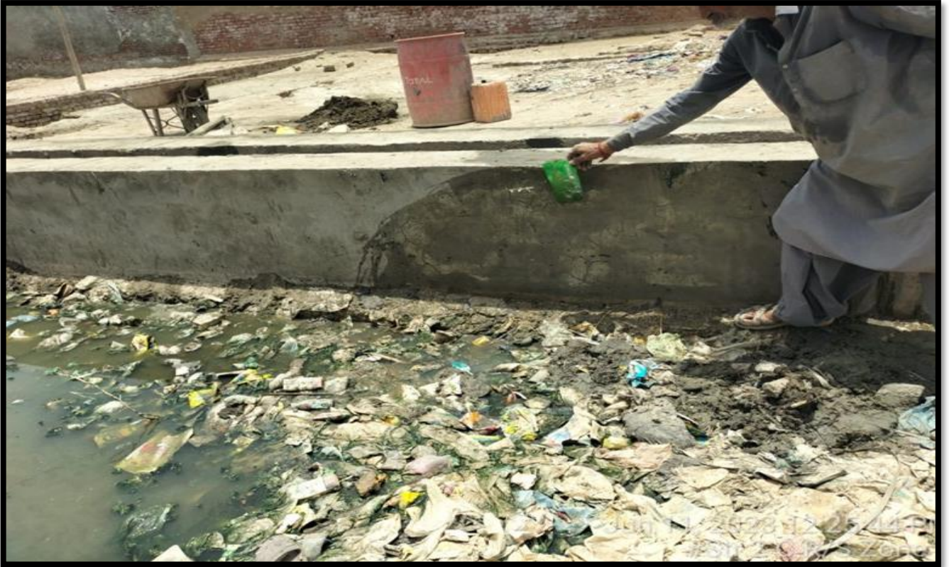
WW-08 (Zone-B) Plaster of Brick masonry Drain at Al Murtaza Colony work is in progress
