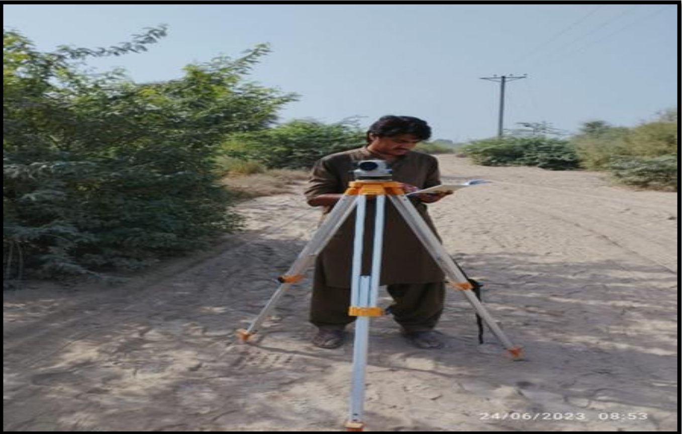
WW-19 During Survey of 500mm diameter Rising Main Aqilpur to Noor Wah work is in progress
