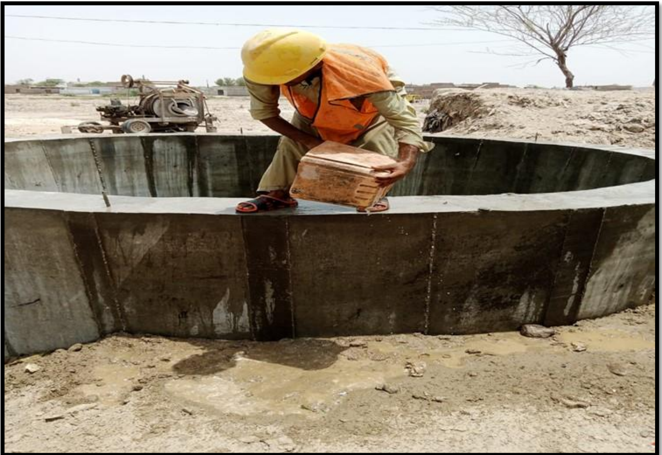
WW-08 (Zone-B) Curing of Sump at Al Murtaza Colony work is in progress
