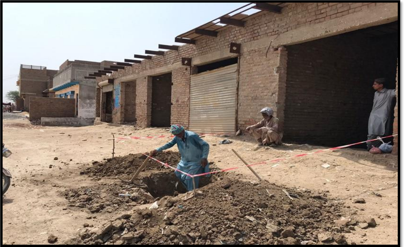
WW-16 Pit for checking utilities at Saddar to Shamb-e-Sha Rising Main route work is in progress
