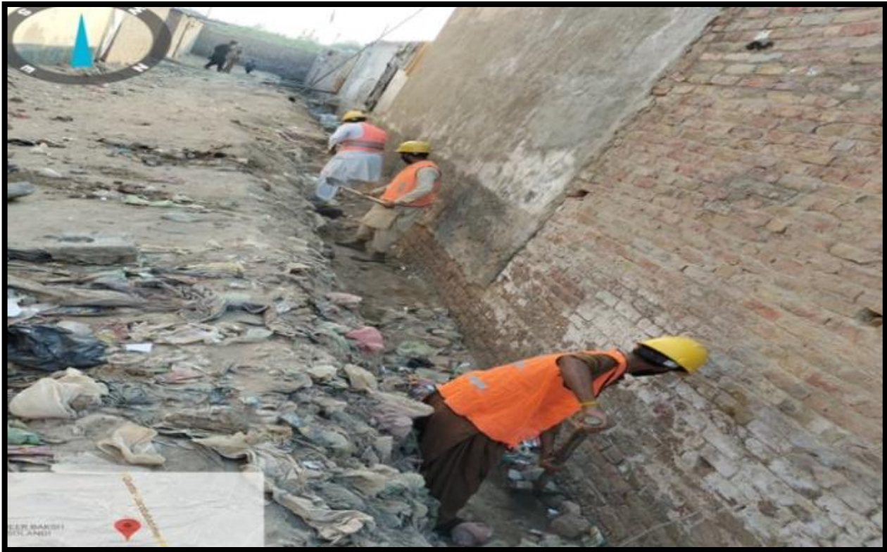
WW-08 (Zone-B) Plaster of Brick masonry drain at Murtaza Colony work is in progress
