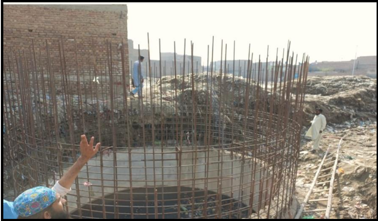
WW-0 (Zone-A) Concrete Pouring work at Phool Bagh is in progress
