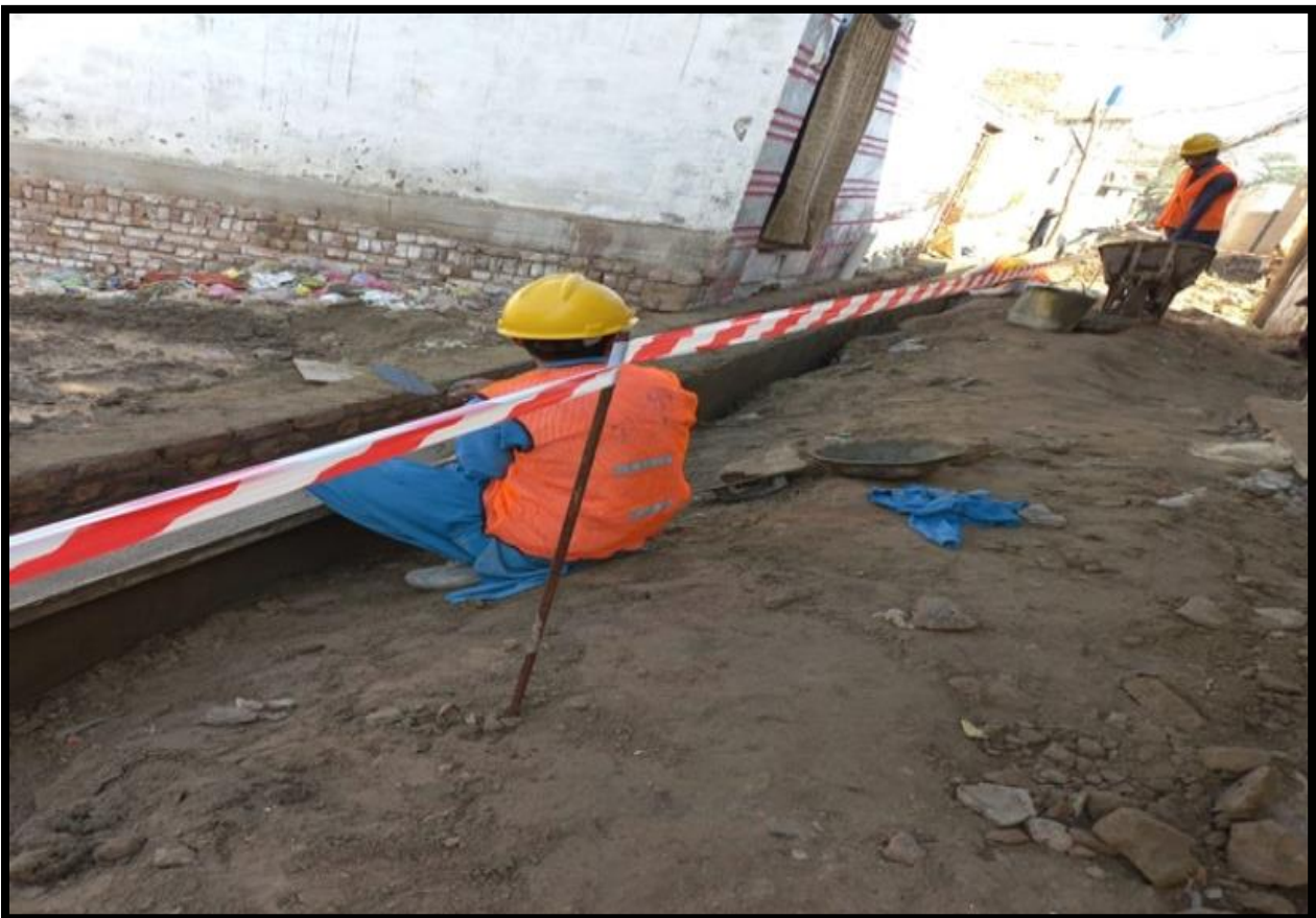
WW-08 (Zone-B) Plaster of Brick masonry drain at Murtaza Colony work is in progress
