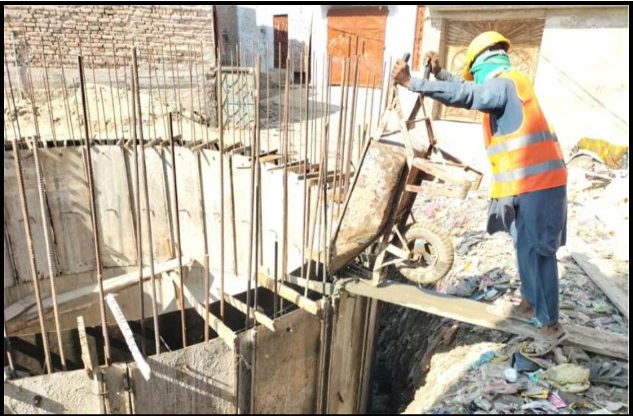
WW-07 (Zone-A) Concrete pouring at Phool Bagh work is in progress
