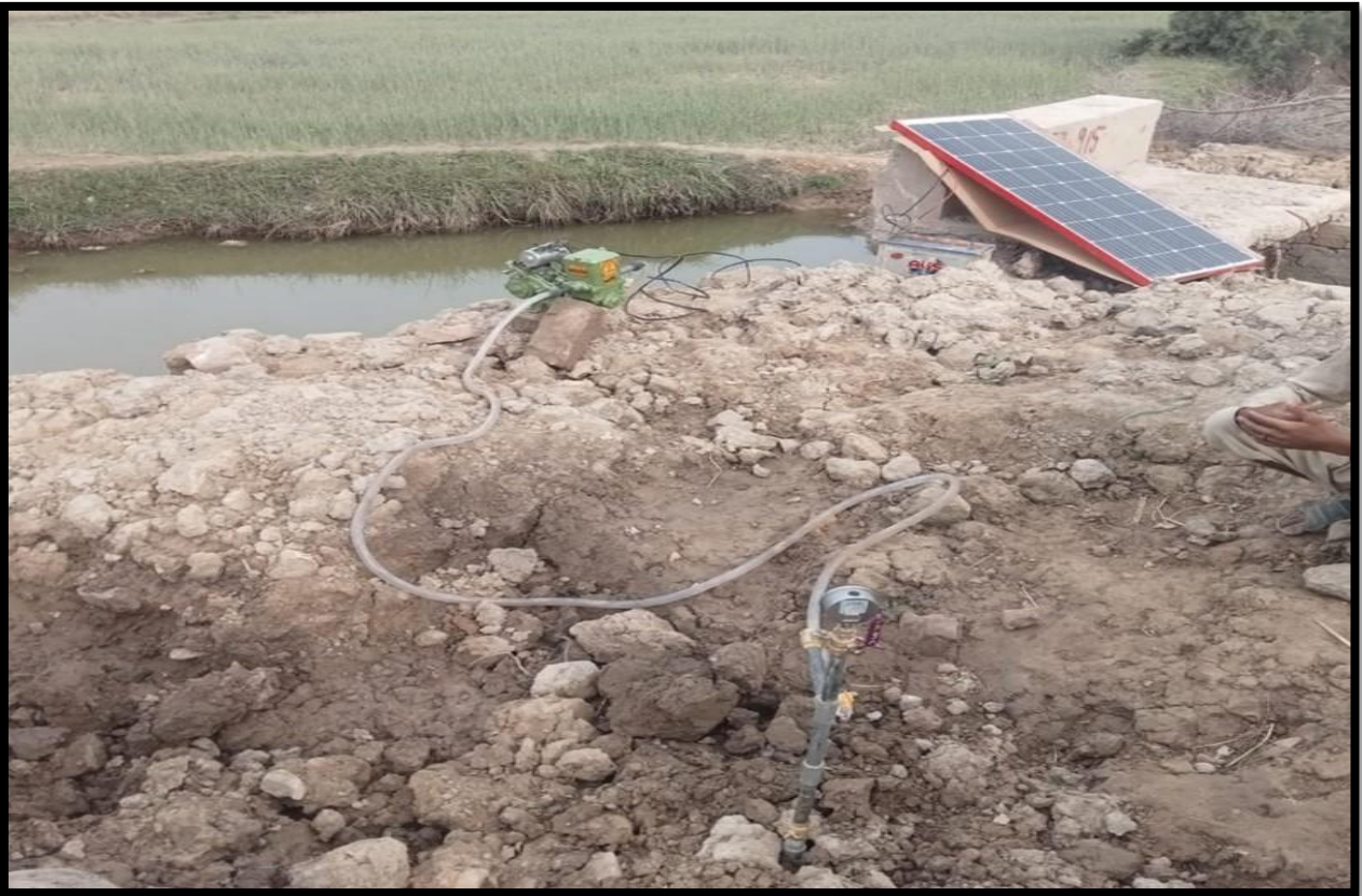
WW-12: Hydrostatic pressure test is in progress
