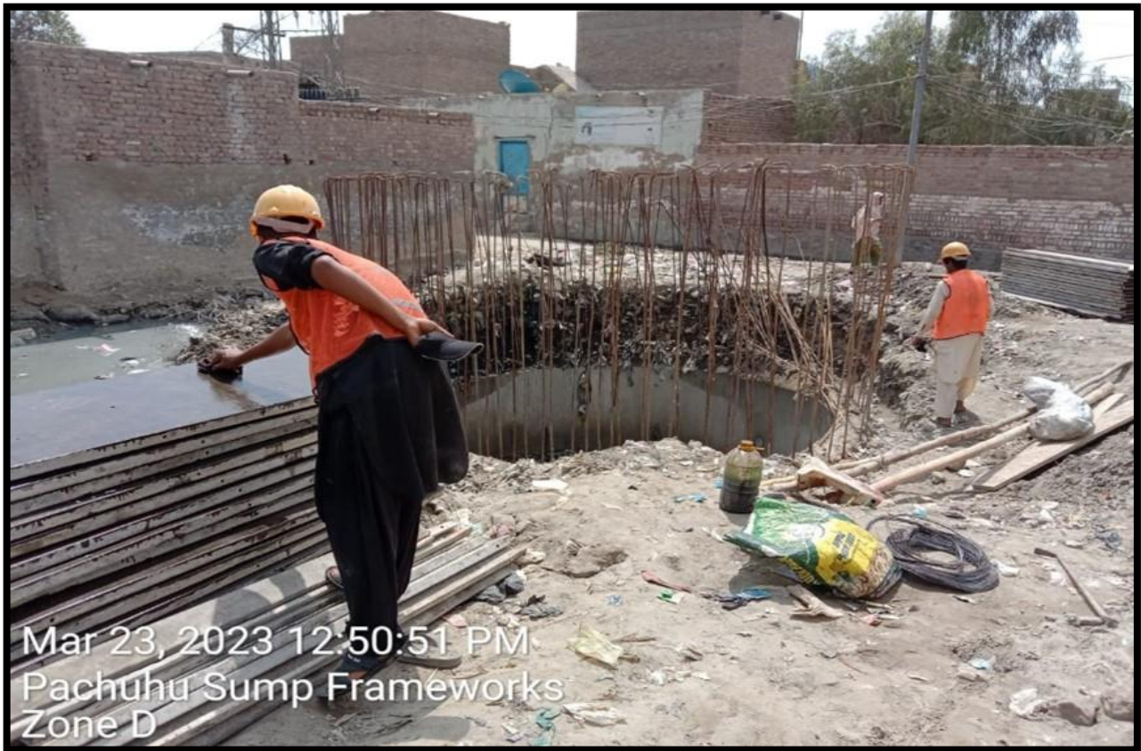
WW-10 (Zone-D): Reinforcement and formwork for Sump work is in progress
