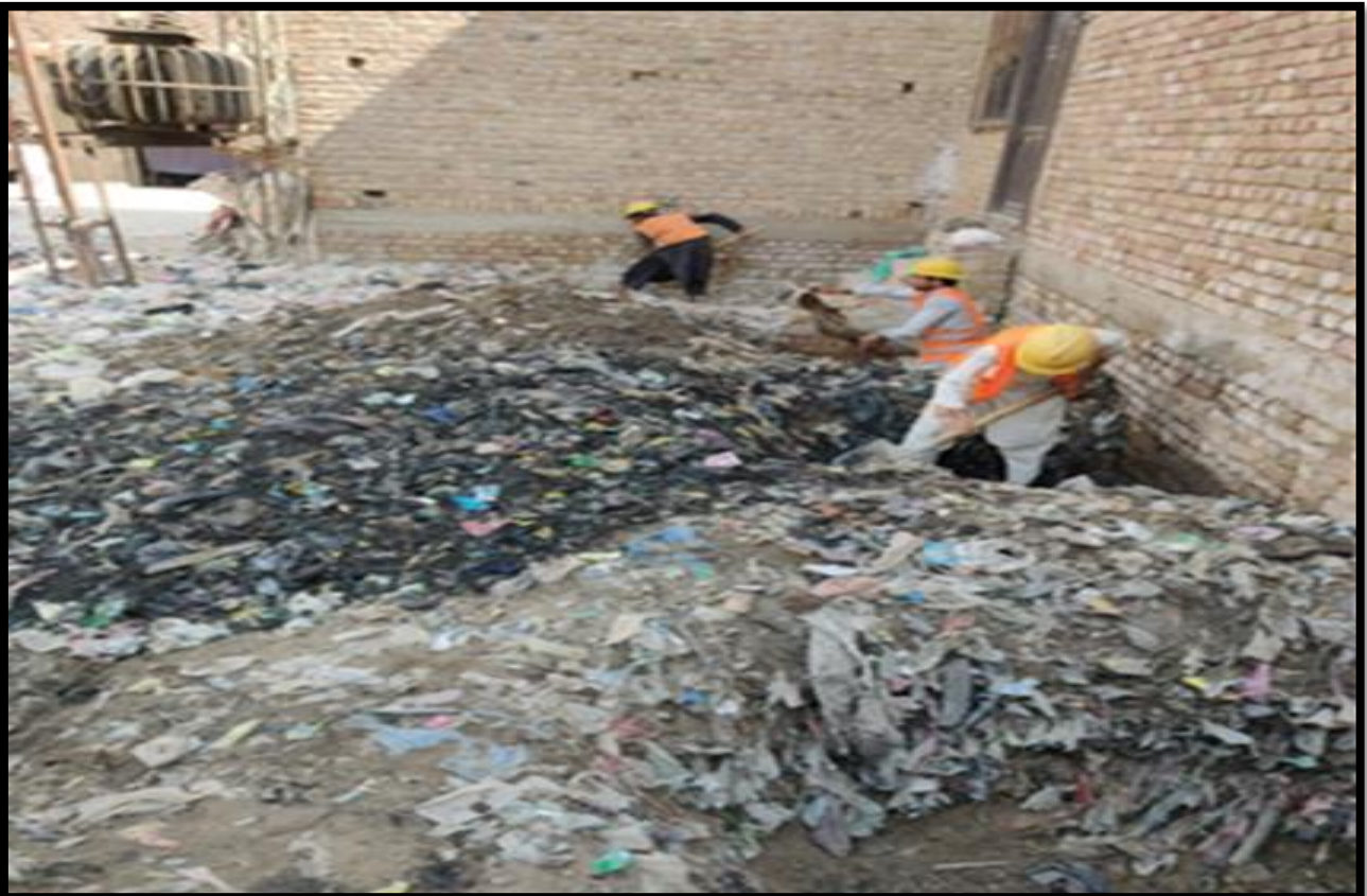
WW-07 (Zone-A): Work in progress at Phool Bagh Sumping Station
