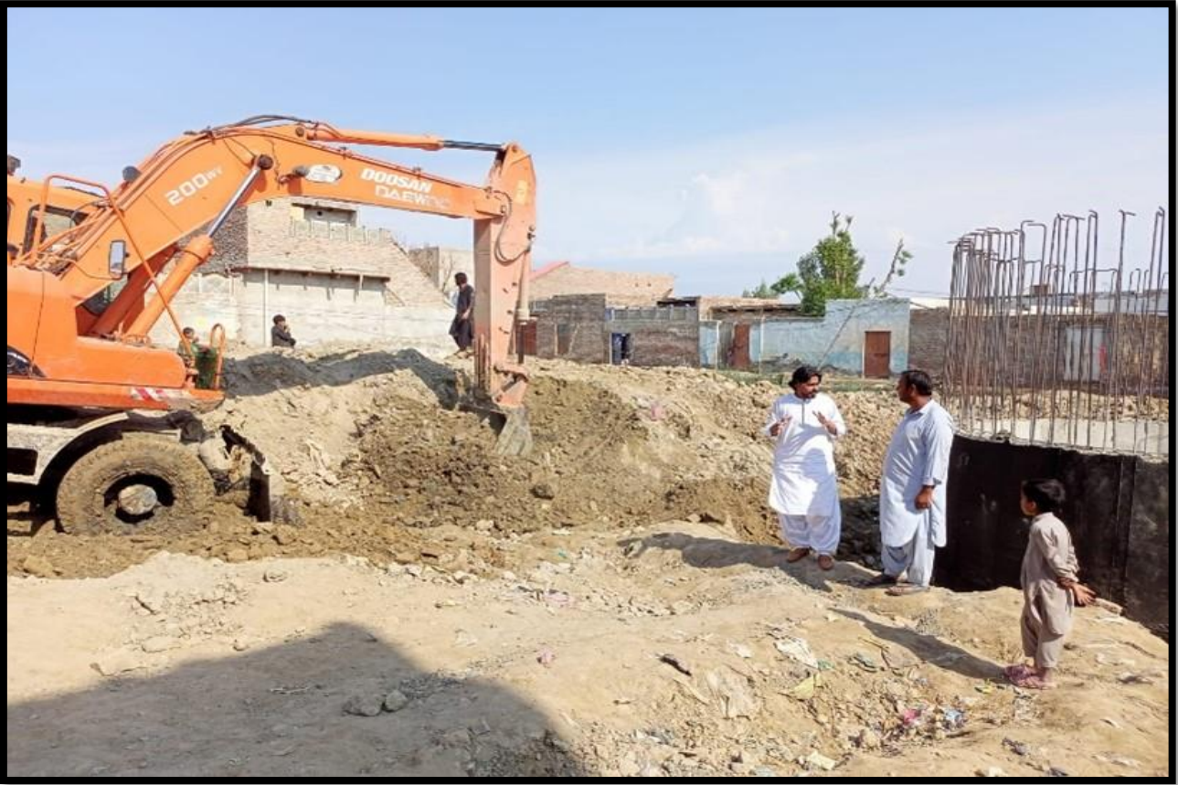
WW-07 (Zone-A): Sump Sinking work is in progress
